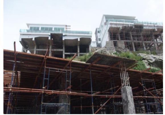
C1 ground-floor formwork with building A5 and A6 in the background
