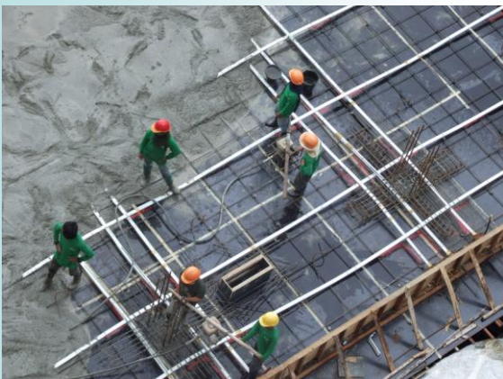
Building A4 superstructure completing 2 nd floor concrete
