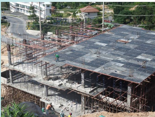
A3 – Completing 3 rd Floor.
