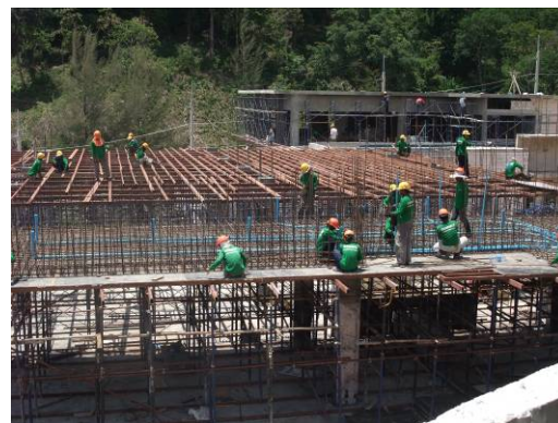
A2 penthouse pool and floor preparation
